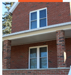
Gil's new windows
