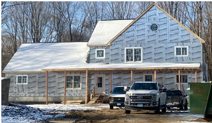
Progress as of January 2025!
