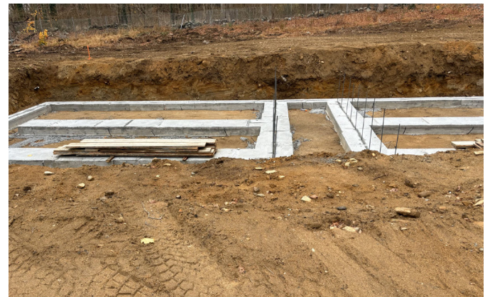
By November, the foundation was set.
