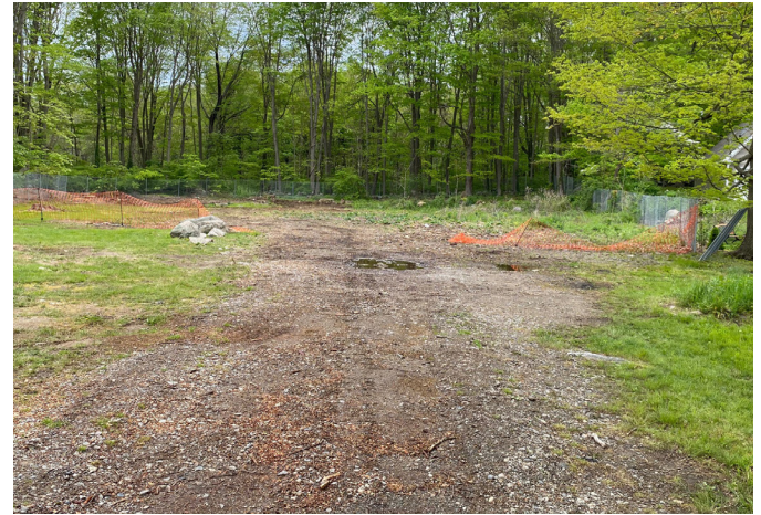
In May 2024, the new building site was leveled.
